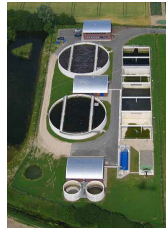
Fig: 1: Aerial photo of the Glückstadt wastewater treatment plant
