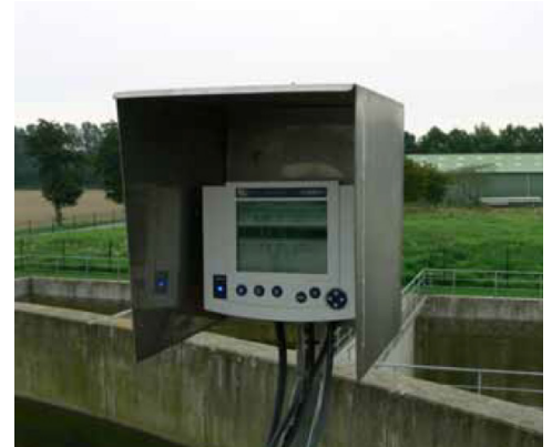
Fig. 3: Ammonium-based control: The new dynamic control acc. to ammonium stops the blowers when ammonium reaches a specific value
